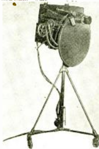
Photo above shows a lighter weight direct pickup for studio use, the photo-cell being placed behind the scanning disc and lens.
